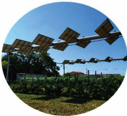
Figure 1 Synergies between crop and photovoltaic panels in agrivoltaic (AV) system
