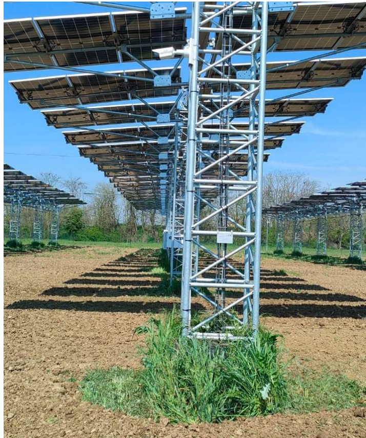
Figure 18. Uncultivated buffer zone in the APV system of Università Cattolica del Sacro Cuore, Piacenza, Italy. The supporting pillars prevent the machines to execute weeding ( Original photograph taken by the authors at the APV plant of Università Cattolica del Sacro Cuore, Piacenza, Italy ).
