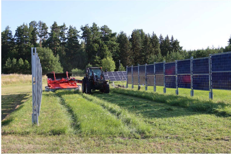
Figure 5. Ley grass harvester in a vertical APV structure facility in Sweden ( Reprinted from [130] with permission of Elsevier ).
