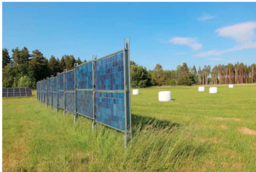
Figure 16. Grass not removed by the forage harvester close to the PV modules support structure (Reprinted from [23] with permission of Elsevier).
