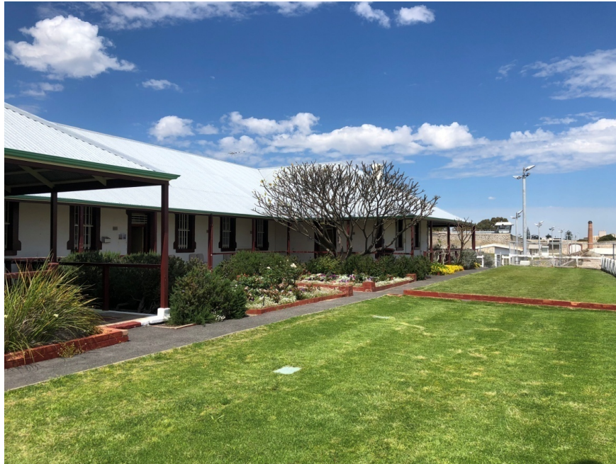
Figure 2: The Literature Centre is located in the former hospital of Fremantle Prison
