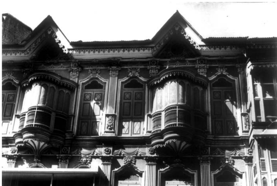
Figure 12.12 The craftsmanship in wooden façades, Siddhpur. Courtesy the author.
