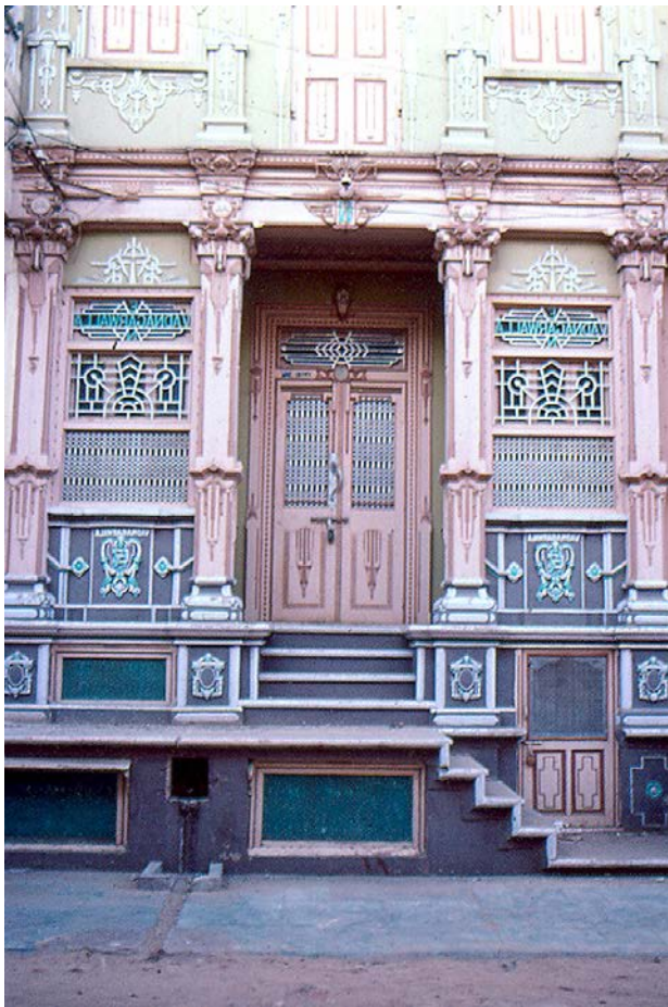
Figure 12.2 A typical Bohra house. Courtesy the author.
