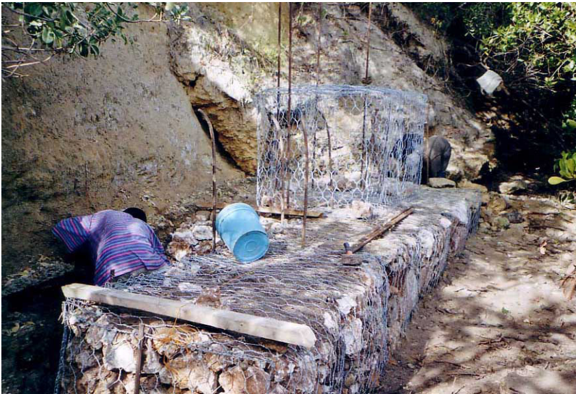
Figure 10.9 Creation of structures to protect against the erosion in the Husuni Kubwa Palace, Kilwa Kisiwani. Courtesy the authors.
