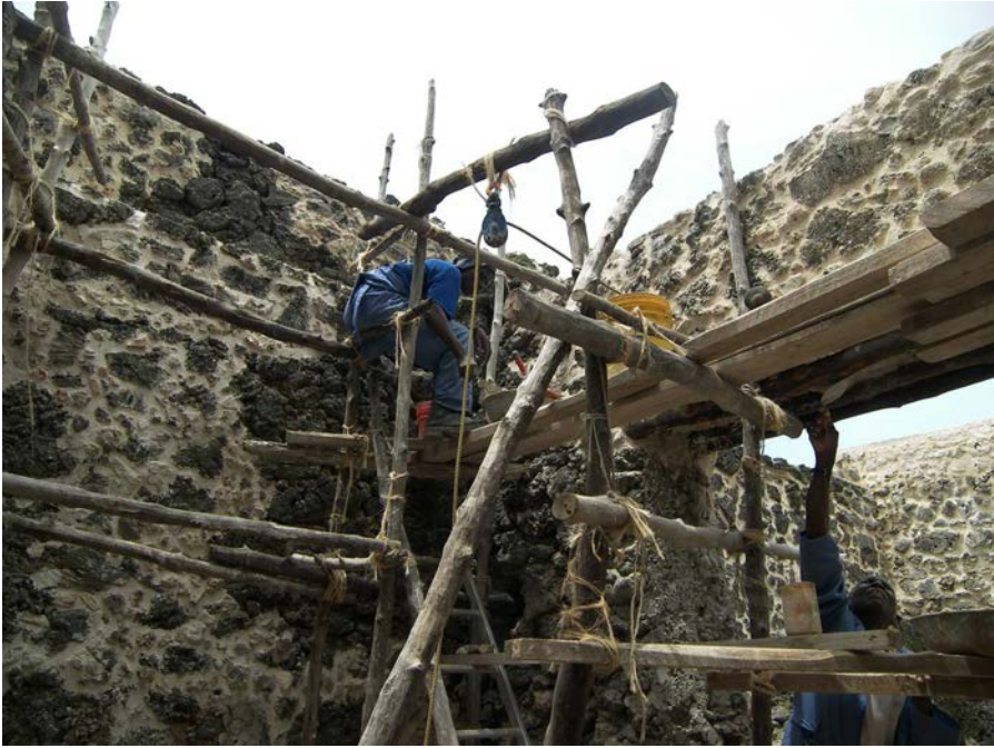
Figure 10.17 Works in progress, Songo Mnara. Courtesy the authors.
