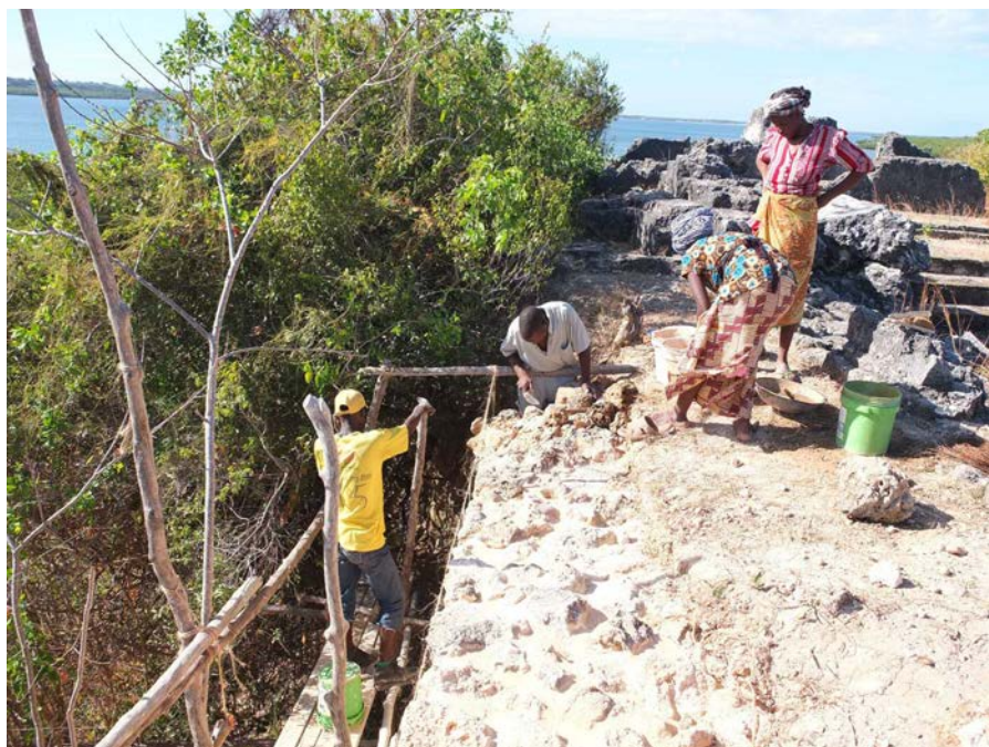
Figure 10.16 Works in progress, Husuni Kubwa, Kilwa Kisiwani. Courtesy the authors.
