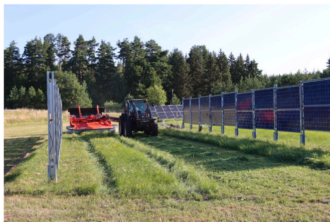
Fig. 3. Vertically mounted APV system during the first cut in 2021 and reference CGMPV system in the background.
